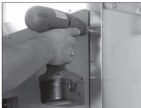
Figure 2.1a - Install unit using all supplied fastening hardware.
