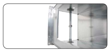
7.3 Validate the orientation of the UV Bio-Wall Max to the air-flow which should be parallel for optimal performance.
