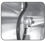
9.3 Connect the cable of the UV Bio-Wall Max to the ballast box Pull the colored wire-set (20 wires) from the UV Bio-Wall Max into the ballast box through the knockout located between the 2 fans and secure the cable connector to the ballast box.
